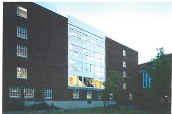
After: New windows
