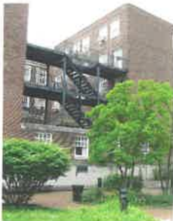
Before: Open egress stairs
